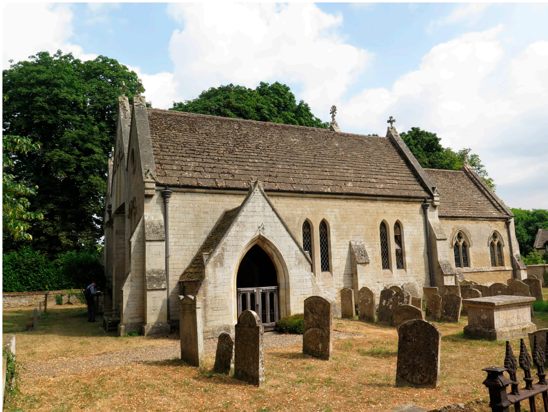
Church of St John the Baptist, Stibbington, Cambridgeshire, constructed of Middle Jurassic Lincolnshire Limestone.
