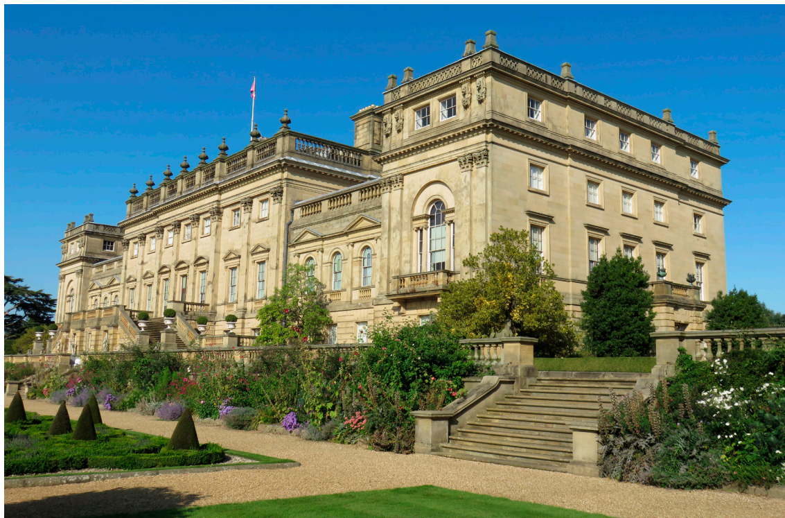
Harewood House, near Leeds, West Yorkshire, constructed of Carboniferous Millstone Grit sandstone.
