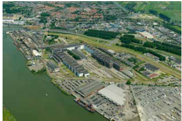
Rod Mill and Wire Processing Centre, Alblasterdam, The Netherlands
