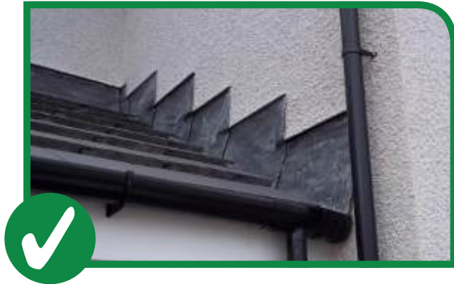
Photo 1 – Example showing flashing linking to cavity trays
